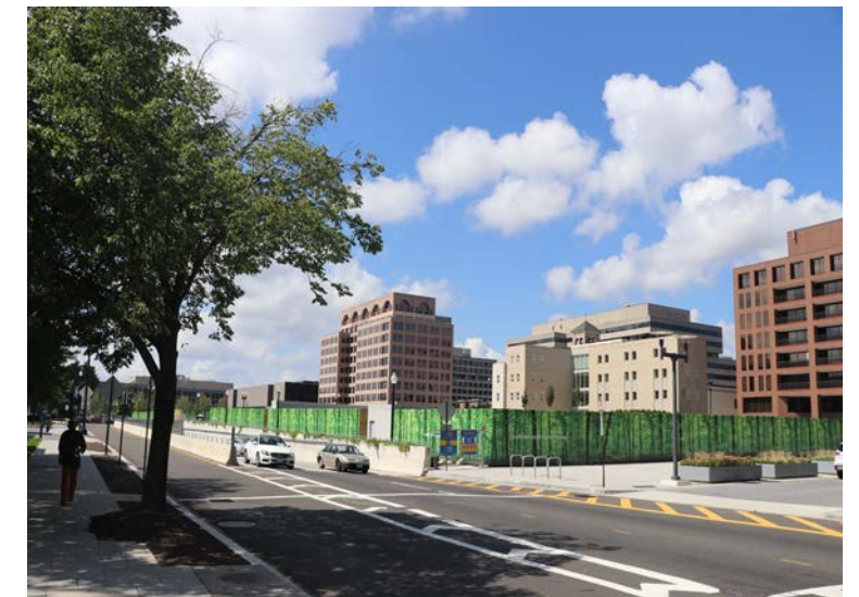
2: EXISTING CONDITION: VIEW OF SECOND STREET SIDEWALK LOOKING SOUTHWEST
